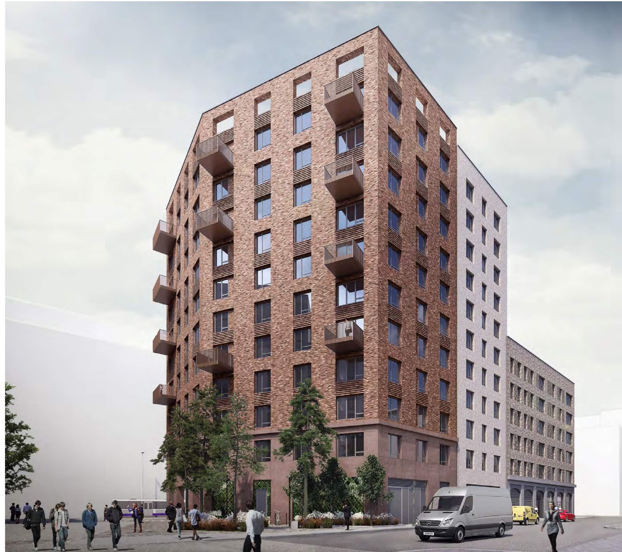
CGI view down New Kingsley Road and Old Bread Street to the west.
